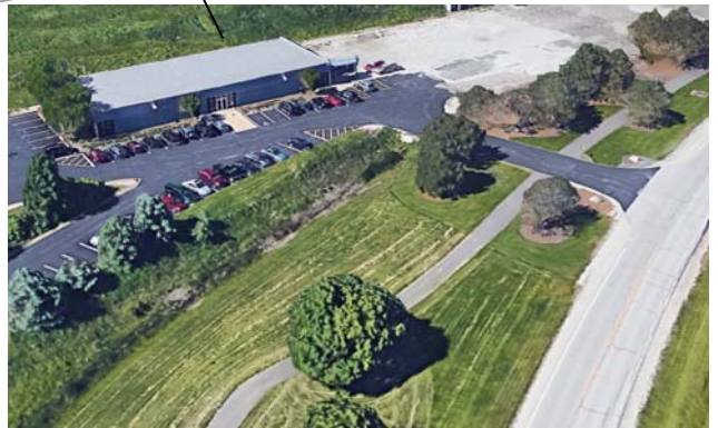
Aerial View of Building
